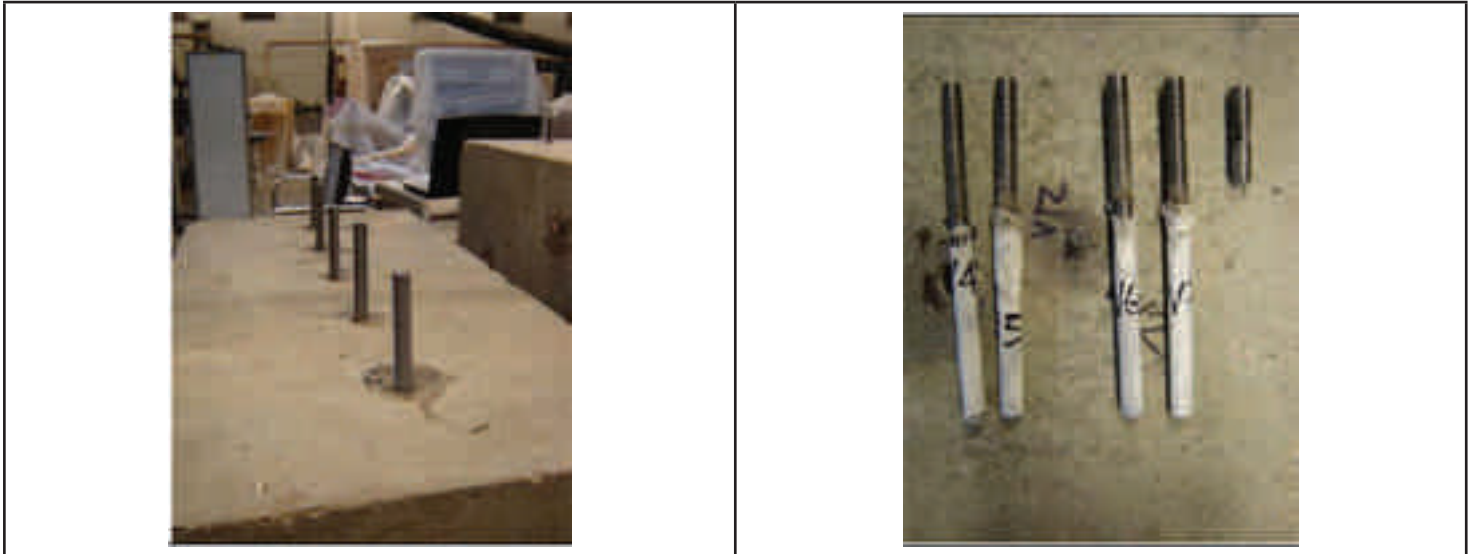
Figure 8.4: - Pull-out failure of Test No. VF8-A1 after tensile loading in dry cleaned holes
